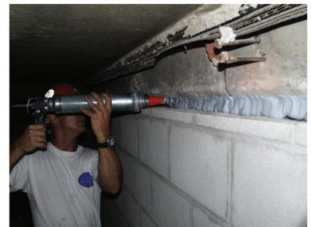
Fire rated sealant being installed to create a rated partition.
